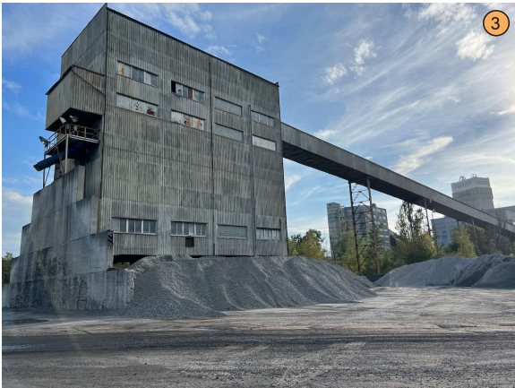
Coal hopper, with conveyor belt over rail line into mine.
